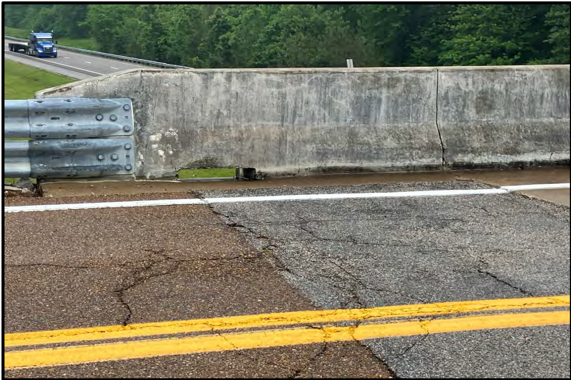
Photo 6: View of bridge draining system from the east side of the bridge.
