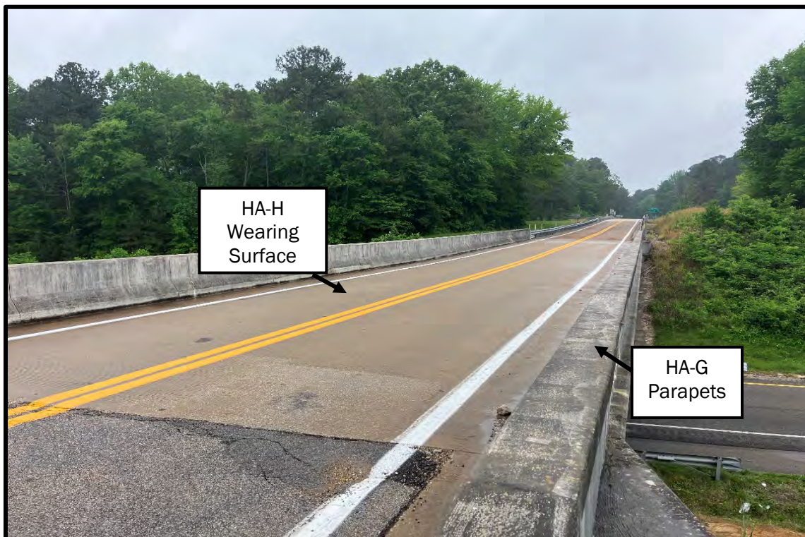
Photo 4: View of HA-G and HA-H from the north end of the bridge facing south.
